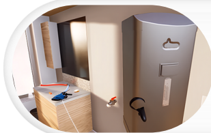
Electric Heater Installation
